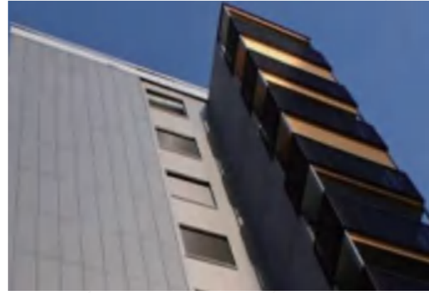
瑞士伯尔尼铜铟镓硒建筑光伏一体化 Swiss Bern Copper Indium Gallium Selenium Building Photovoltaic Integration
